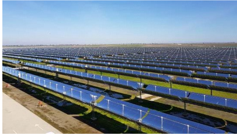
CSP (Concentrated Solar Power) Asset (Lebrija)
