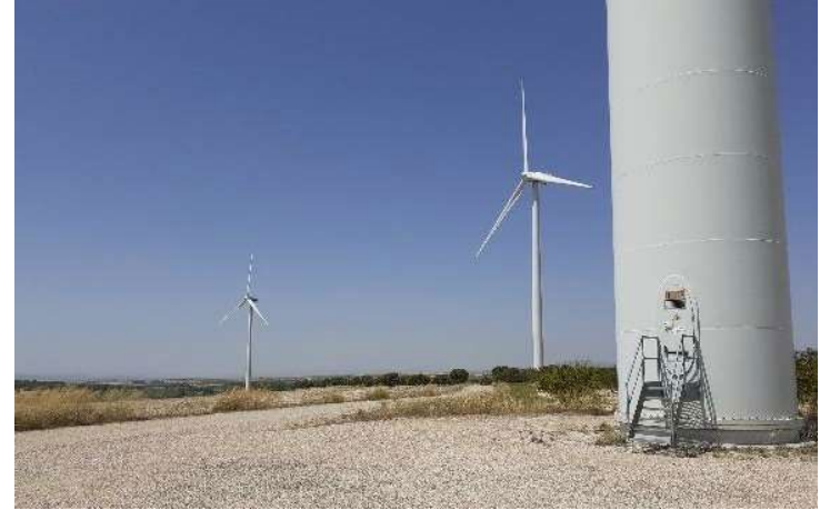
Tella wind farm (50 MW) located in Murica (east coast of Spain, south of Madrid)
