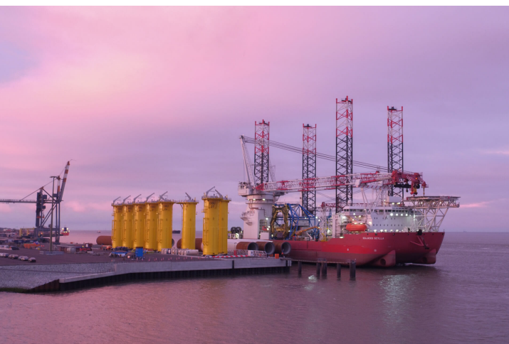
The installation vessel transported three monopiles and transition pieces per trip from the port of Cuxhaven to Deutsche Bucht's offshore site in the German Economic Exclusive Zone.
