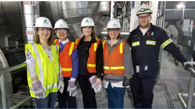
The Payroll team taking a tour of our 260 MW North Battleford thermal facility located in Saskatchewan.
